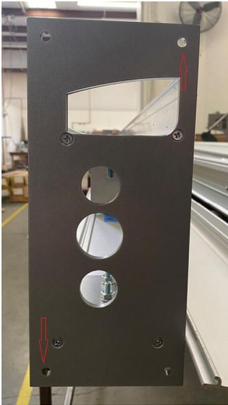
Place the horizontal rail(s) at predetermined height above the finished floor. The attached column brackets should be against the building wall in the correct position aligned with services. Attach the column brackets to the building wall using the four (4) pre-drilled holes in the column brackets.
